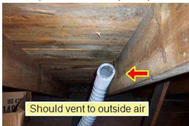
9.4 Picture 1 Exhaust from bath fan
