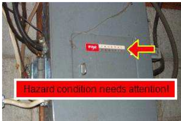
7.2 Picture 1 Federal Panel in basement
